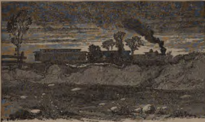
A Marl-Bed on the Line of the Chesapeake and Ohio Railroad.
